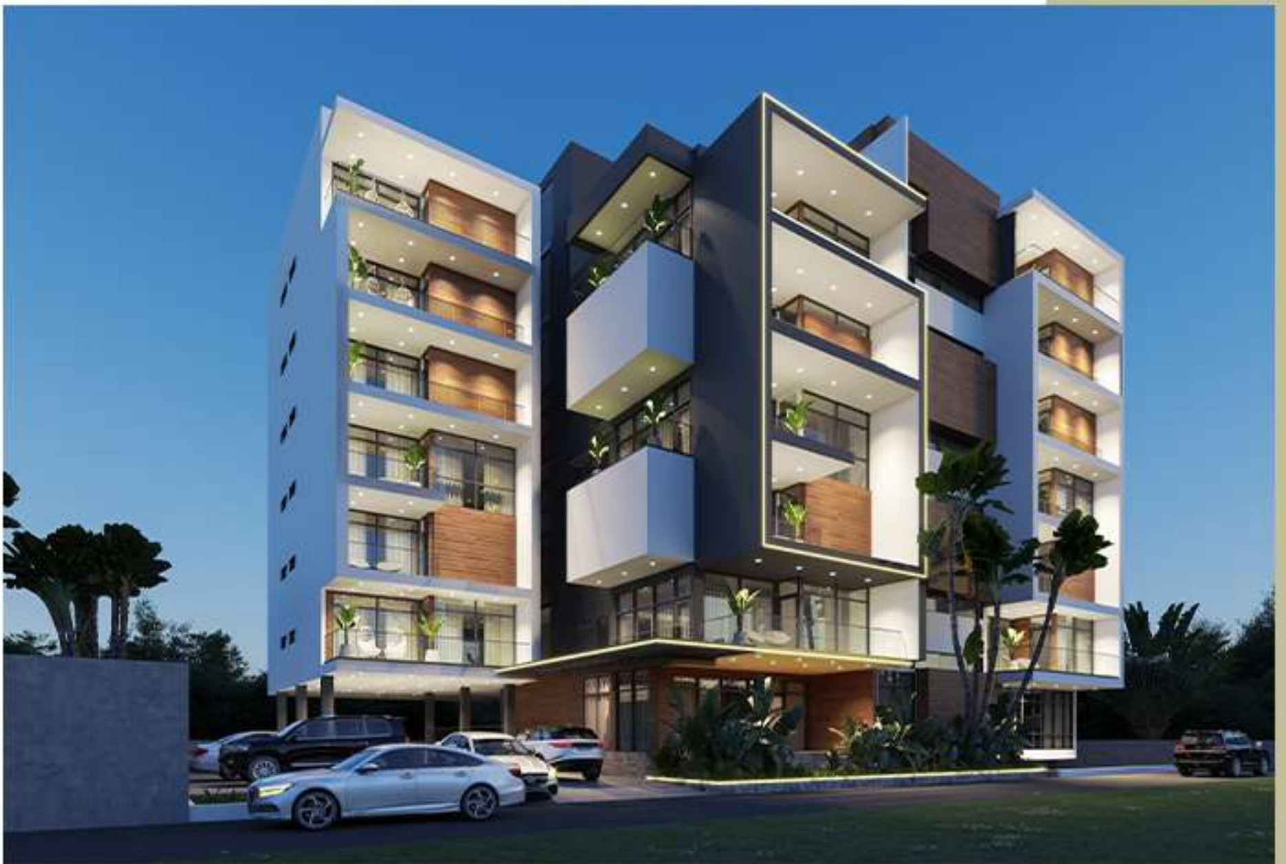
6 Storey Luxury Apartment building, at Kaneshie, Accra
